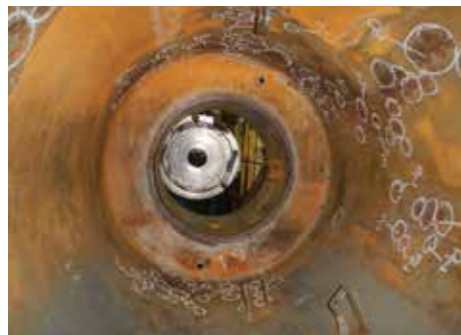
Condition prior blasting, application of coatings and installation of EIMag
