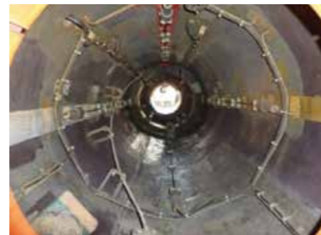
Condition after 5 years with EIMag in continuous operations
