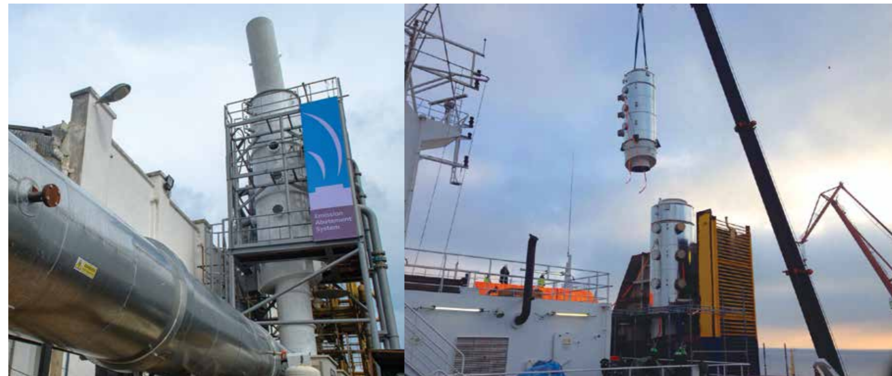
Purpose-built EGCS Testing Facility
